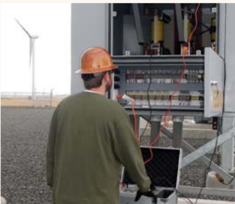
Finley Ledbetter III of Vacuum Interrupters, Inc. uses magnetron atmospheric testing to identify faulty interrupters in the field without removing the interrupters from their enclosures. Before the portable MAC-TS4 series of test systems with flexible magnetic coils, predictive tests only were conducted at the factory. Field technicians were limited to HiPot pass/fail tests and contact resistance testing, neither of which can predict the remaining life of vacuum interrupters in the field.
