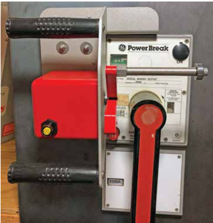
Figure A – RSK-GEPB1 installed on breaker
